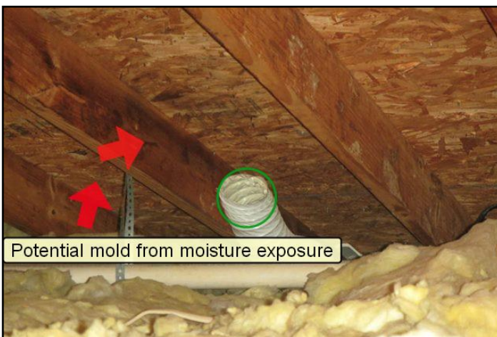
Poor termination location
