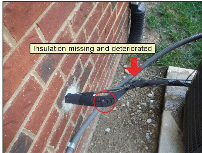
Missing insulation
